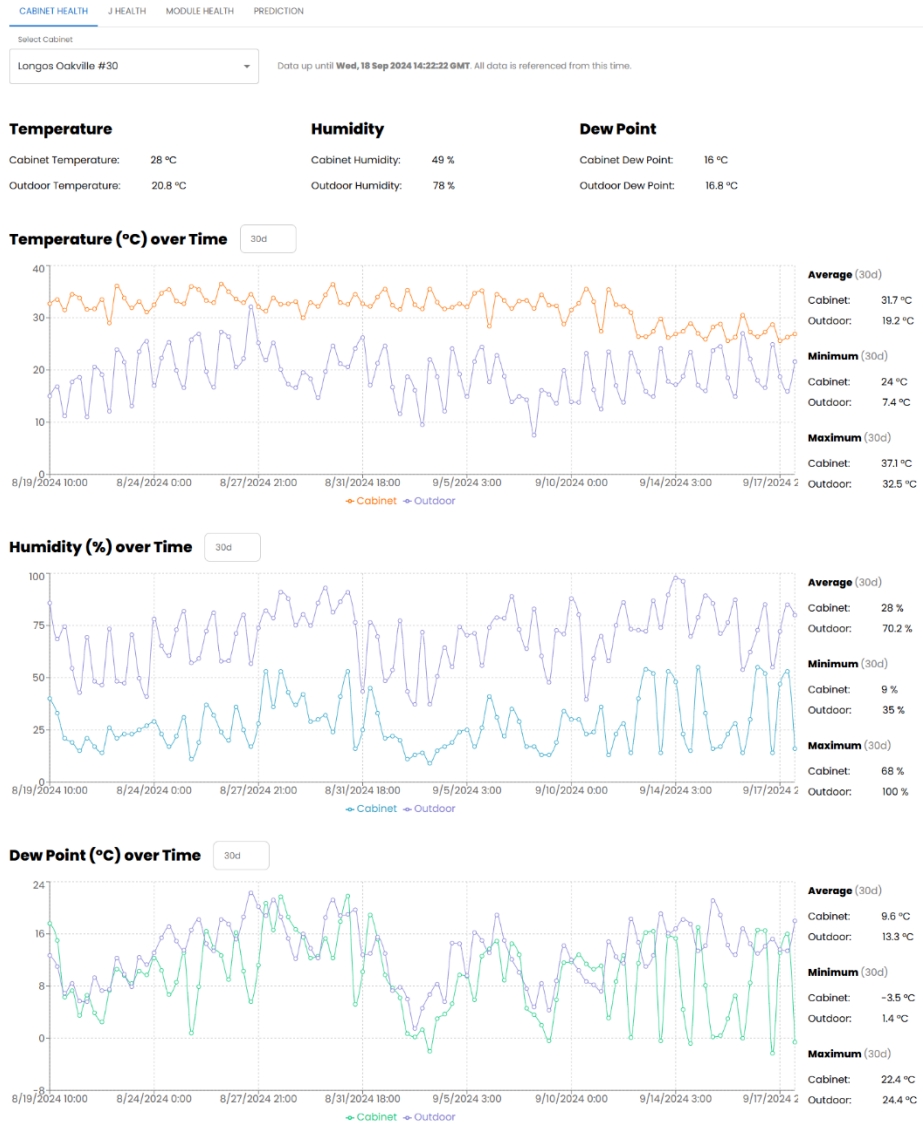
Figure 16. Charging station cabinet health overview shown in eCamion Dashboards
