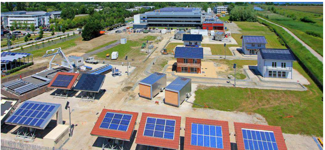
INCAS platform from CEA - a full scale test facility including 4 PASSYS test cells, 4 experimental houses and 10 PV-integration benches
