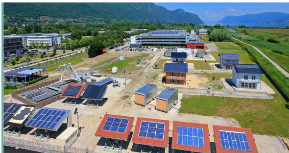
INCAS platform from CEA - a full scale test facility including 4 PASSYS test cells, 4 experimental houses and 10 PV-integration benches
