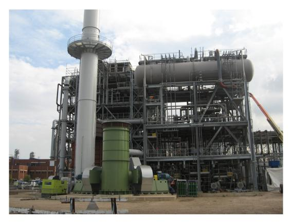
Industrial Boilers are direct-fired boilers designed and used to provide steam to industrial processes. They may use various type of fuels, liquid or gaseous, according to the application. An Industrial Boiler is generally made up of two major systems. One system is the fuel-air-flue gas system (fireside) and the other is the water-steam system (waterside). Heat is provided to convert water into steam.
