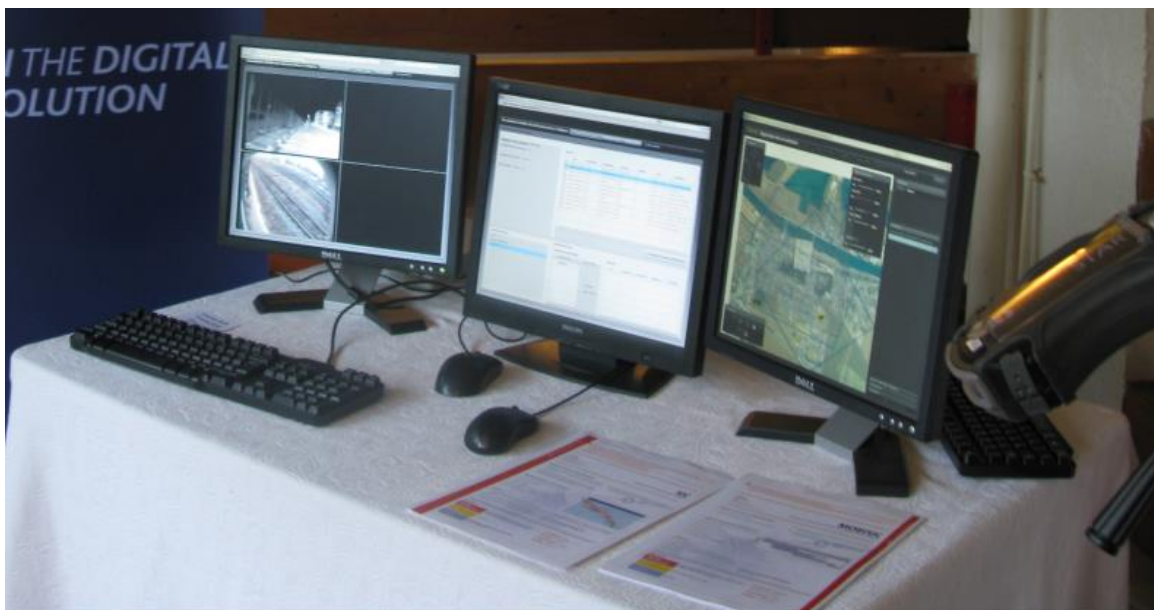
Figure 3.1.1-1 MOBISIC supervision control station
